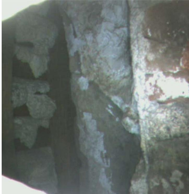
Figure 5: View from scope showing both masonry back-up (to right) and plaster and lathe back-up (to left).
